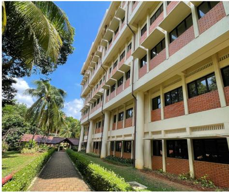
north side where classrooms are located. The glazing materials used is 6mm clear glass with windows size with the area of 1.38m<sup>2</sup> and 2.07m<sup>2</sup> for each opening. The investigation is conducted for floors two to five where classrooms are located along the corridors. This study separates the classroom areas between the north and south facing parts of the building to understand the different illuminances of each area (Fig. 3).
