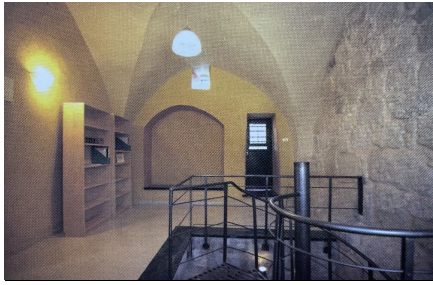
Spiral staircase opening on the first floor before interventions by a user in building 1 (Benelli 2017)
