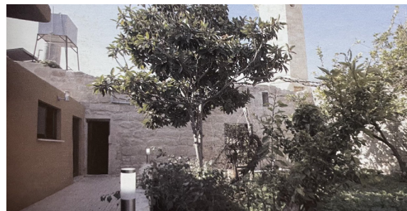
Window on the right side of the façade before dismantling it and replacing it with a door in building no 1 (backyard)
