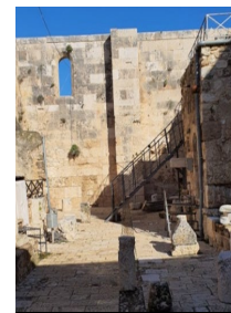
A new iron stair was added by the user building no 1
