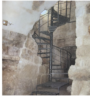
The spiral stair was installed in restoration building 1 (Benelli 2017)
