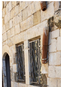
6: Removing Water pipes (clay) in the alley no4
