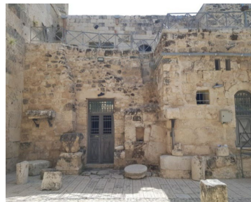
Before interventions by user building no 1
