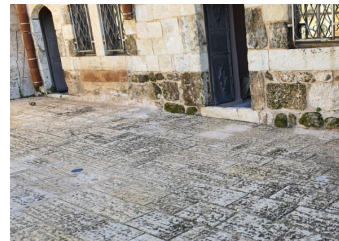
After interventions: removal of the planters building 1
