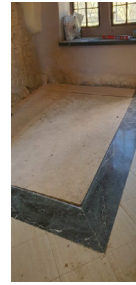
After interventions: Closing the opening of the spiral staircase in building 1
